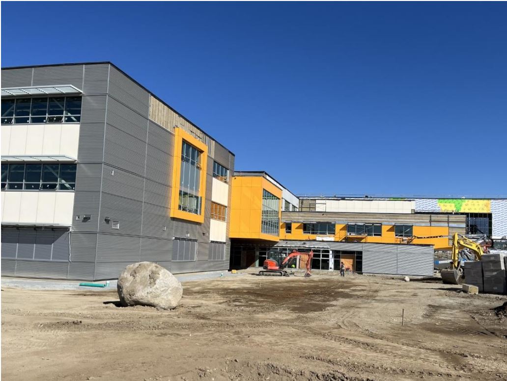
Burnaby North Secondary Replacement
