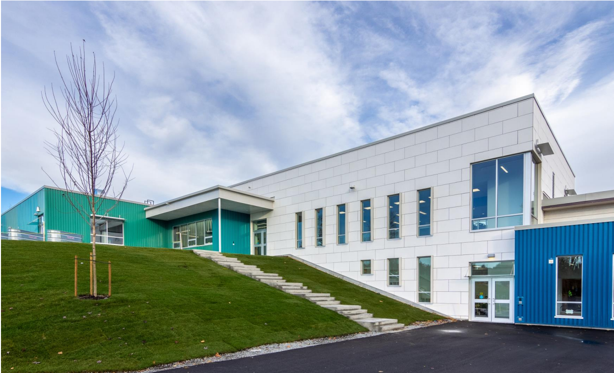
Ecole Parkcrest Elementary – Partial Replacement – new wing
