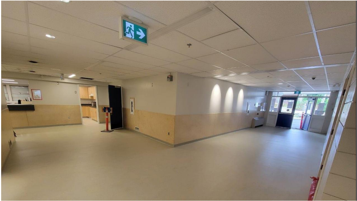
Seaforth Elementary – Seismic Strengthening – interior upgrade
