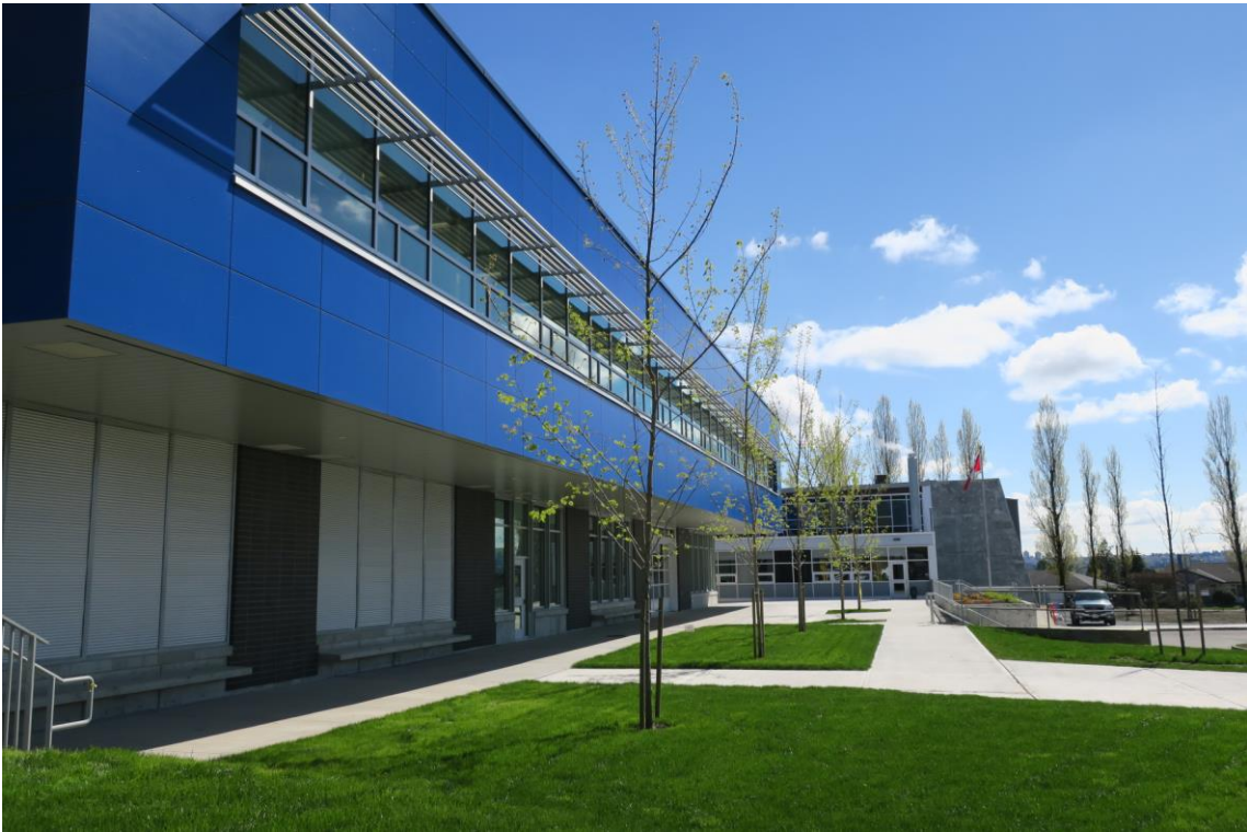
Alpha Secondary School – New Wing (Seismic Partial Replacement)
